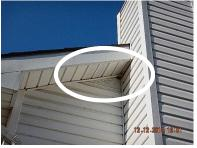
2. Soffits/Fascia/Trim: Aluminum/vinyl covered - -Some loose/missing trim noted. Securing or re-installing may be needed in some areas.
